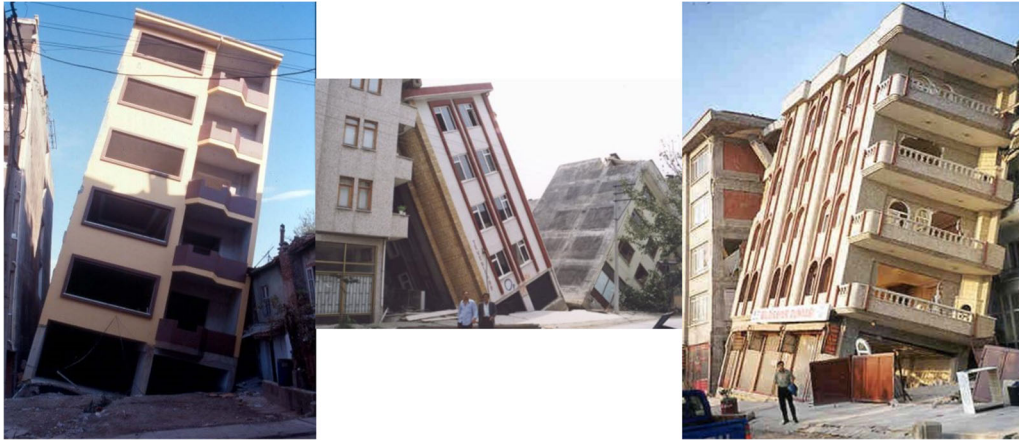
Figure 2.27 Unintended plastic hinging in soil foundations and intact tilted buildings in 1999 İzmit earthquake (Turkey) (Yılmaz et al., 2004; Bird and Bommer, 2004; Anastasopoulos et al., 2010)
