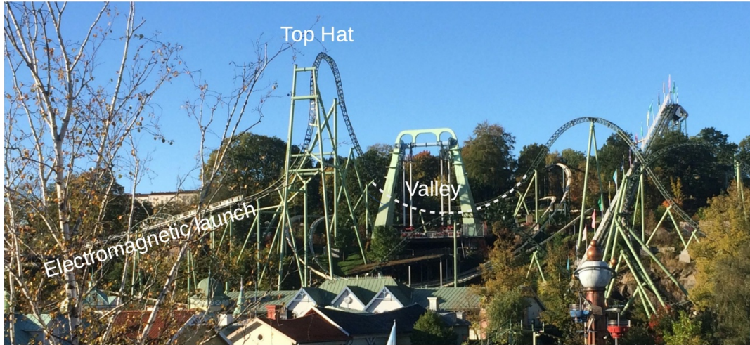
Figure 1. The second electromagnetic (LSM) launch of the Helix roller coaster, followed by an inverted Top Hat and a large valley.
