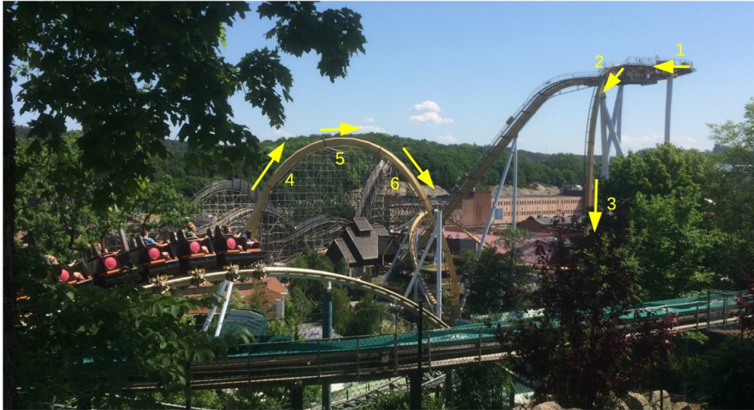
Figure 10. A view of the Valkyria dive coaster together with the inversion following the valley. The yellow arrows indicate the direction of the train, starting with a panoramic tour of the Liseberg amusement park at the top of ride (1), a brief hold looking down (2) before the dive (3) into the an underground tunnel. The train then emerges from the underground tunnel to the left (4) and moves to the right, upside down over the hill (5) and the down on the other side (6).
