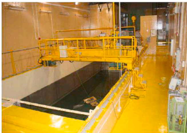
Fig. 6. Spent fuel pool in the Serpong ISSF.
