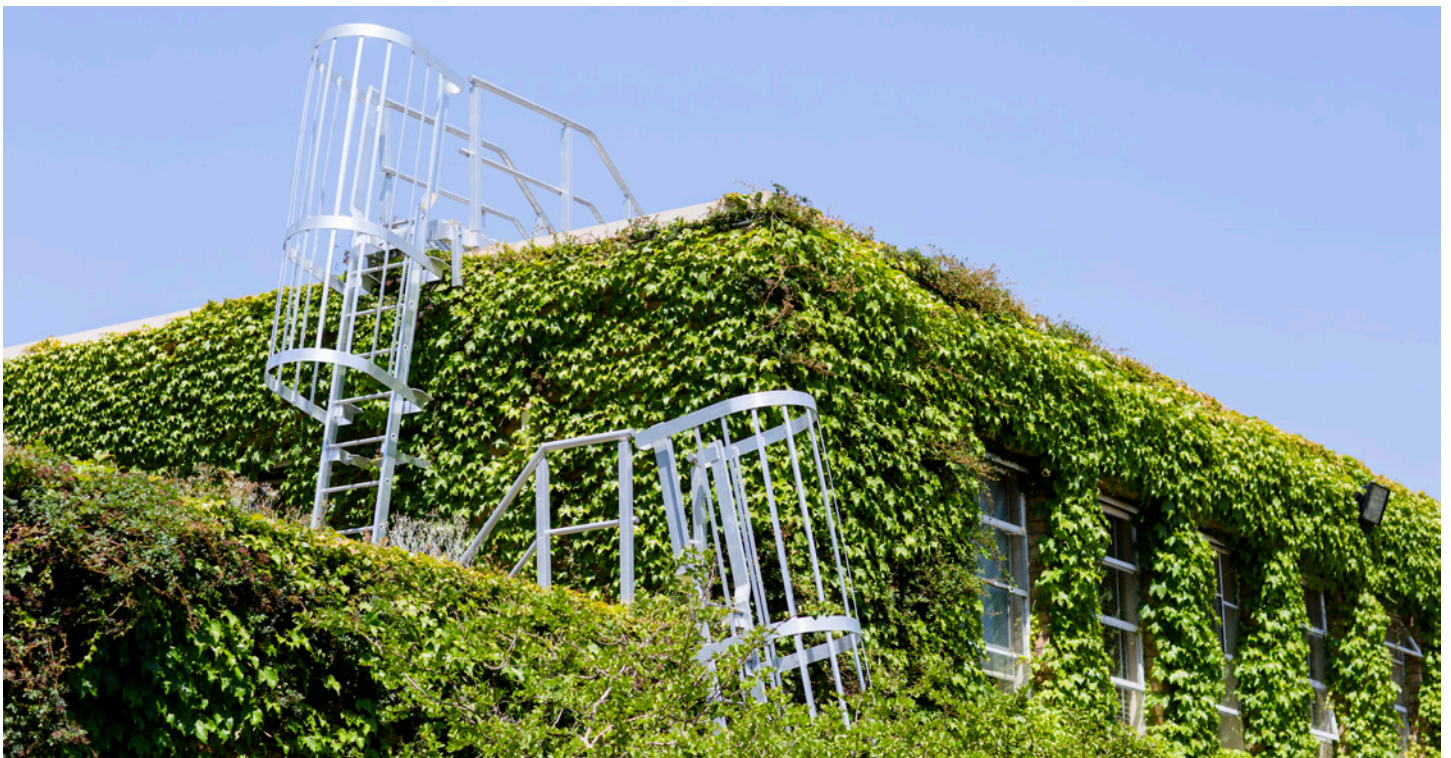
Figure 1. Building Facade. Photograph University of Melbourne
