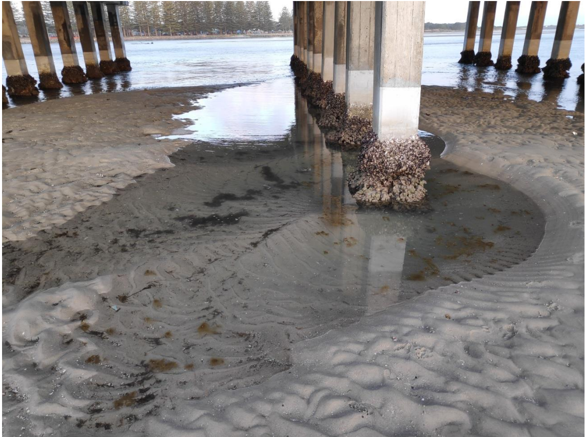
Figure 2.2. Local scour around bridge piers (taken by the candidate)
