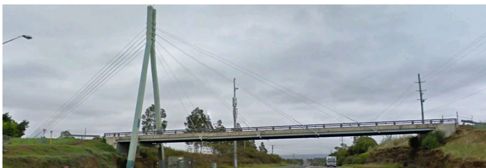
(a) The cable-stayed bridge
