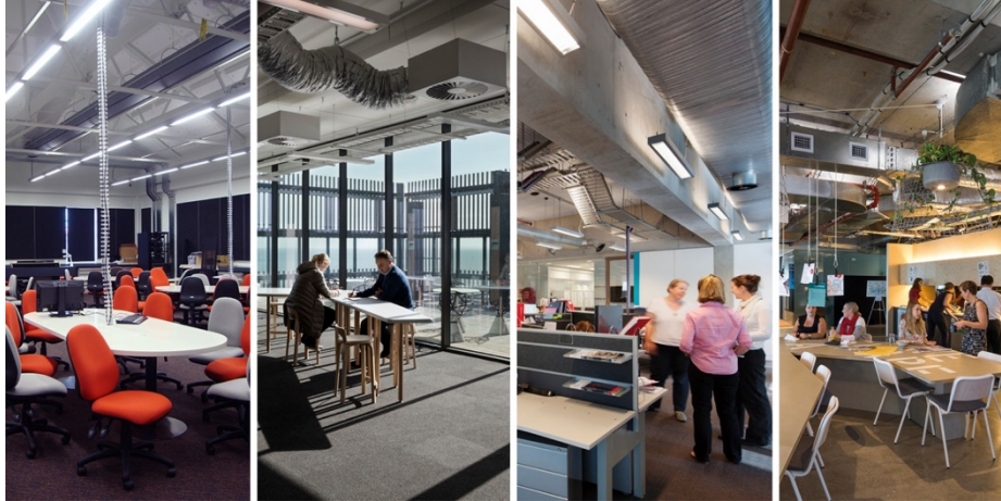
Fig. 2. Existing ductwork systems (left to right). Flexi, rigid, spiral-wound and fabric ductwork.
