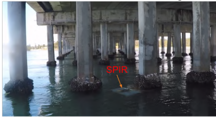
(b) SPIR in Windang bridge
