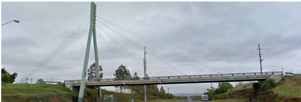
(a) The cable-stayed bridge
