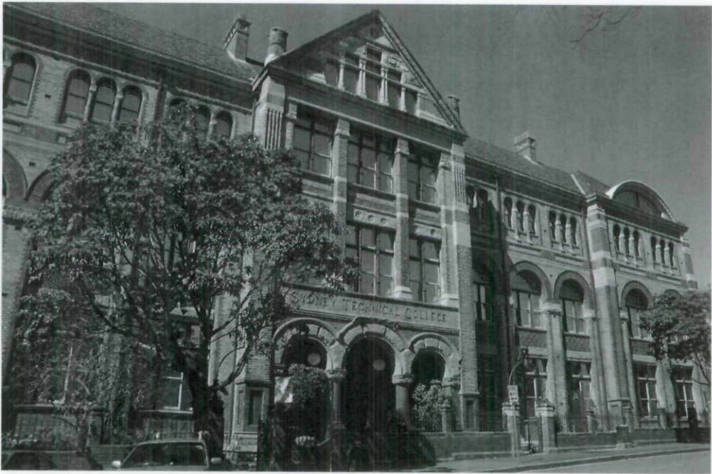
Figure 2: Sydney Technical College (1891), designed by William E. Kemp. Photograph by Kirsten Orr.
