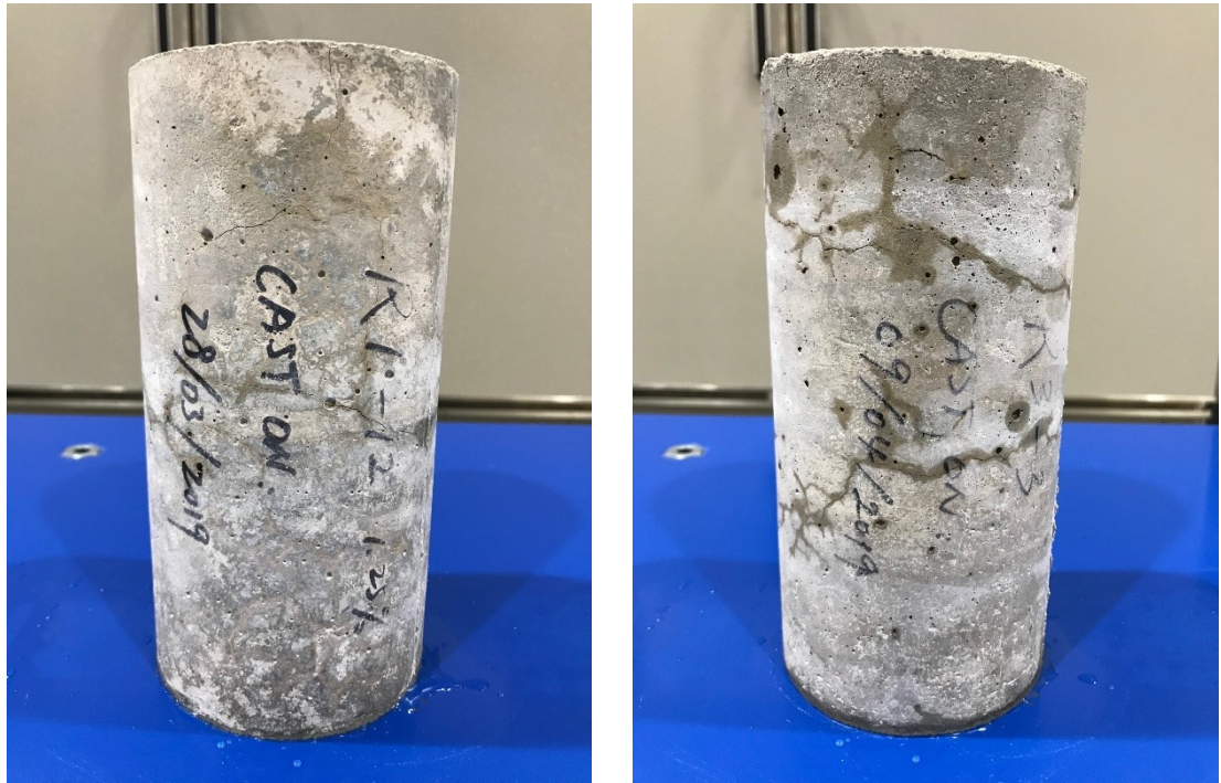
Figure 7. 22 External cracks on cylinders at the age of 500 days, immersed in water and stored in 38 °C climate chamber, without autoclaving specimens
