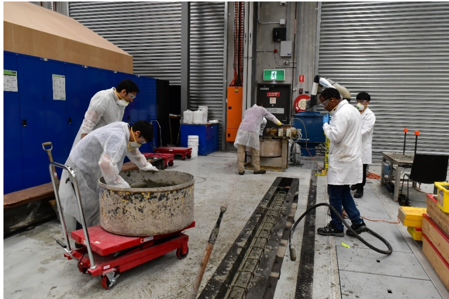
Figure 7. 5 Concrete placement for reinforced concrete beam
