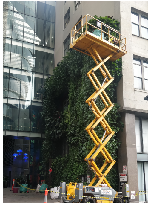
(b) UTS Building 10
