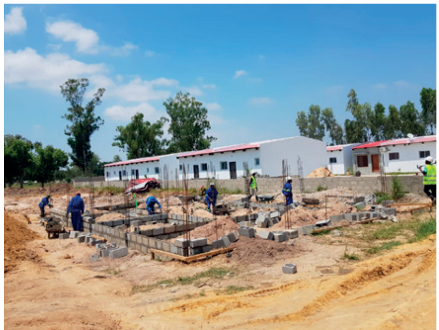
FIGURE 4 Casa Real affordable housing development in Beira, Mozambique
