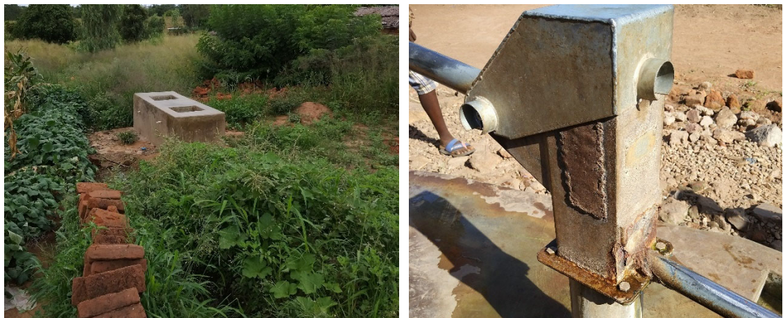
Figure 21: Laundry area in Nkhumba and evidence of continued rusting in Nanchopwa due to saline ground water
