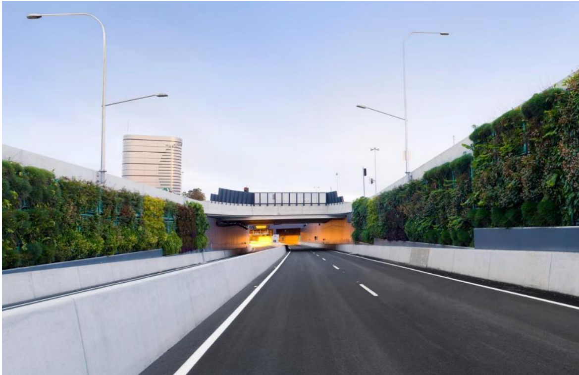
Figure 8 Brisbane Airport Link Cut and Cover
