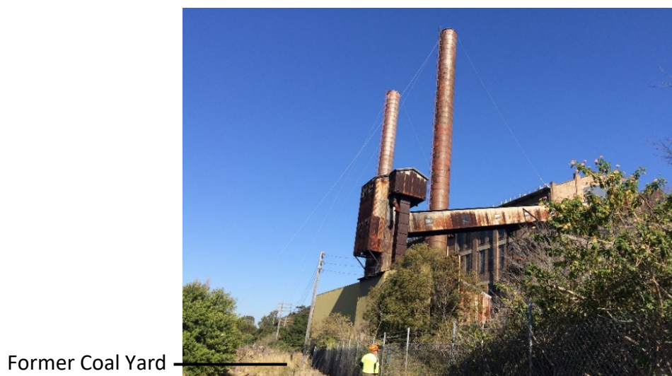
Figure 6.4. White Bay Power Station from a northern aspect of the garden prior to planting.
