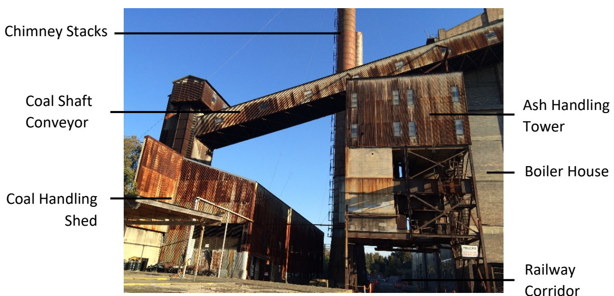
Figure 6.2. Features from the northern aspect of White Bay Power Station.
