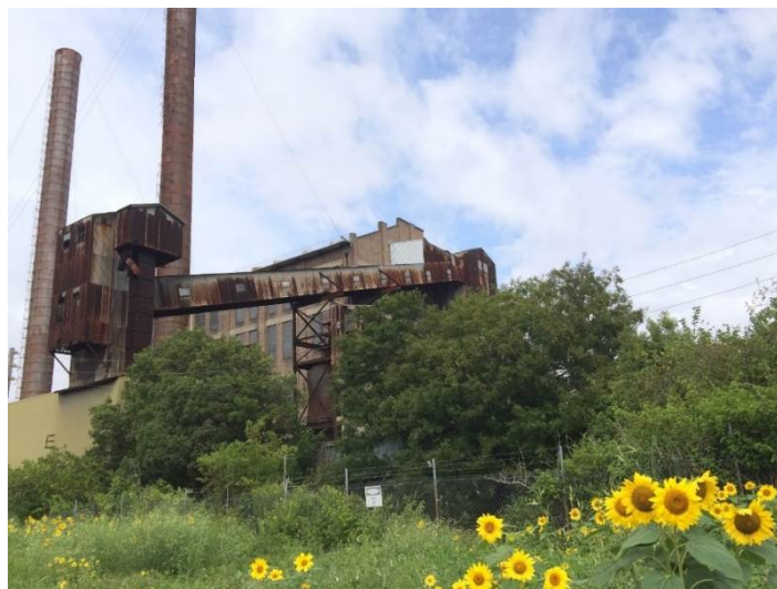
Figure 6.19. White Bay Power Station with phytoremediation garden in the foreground.
