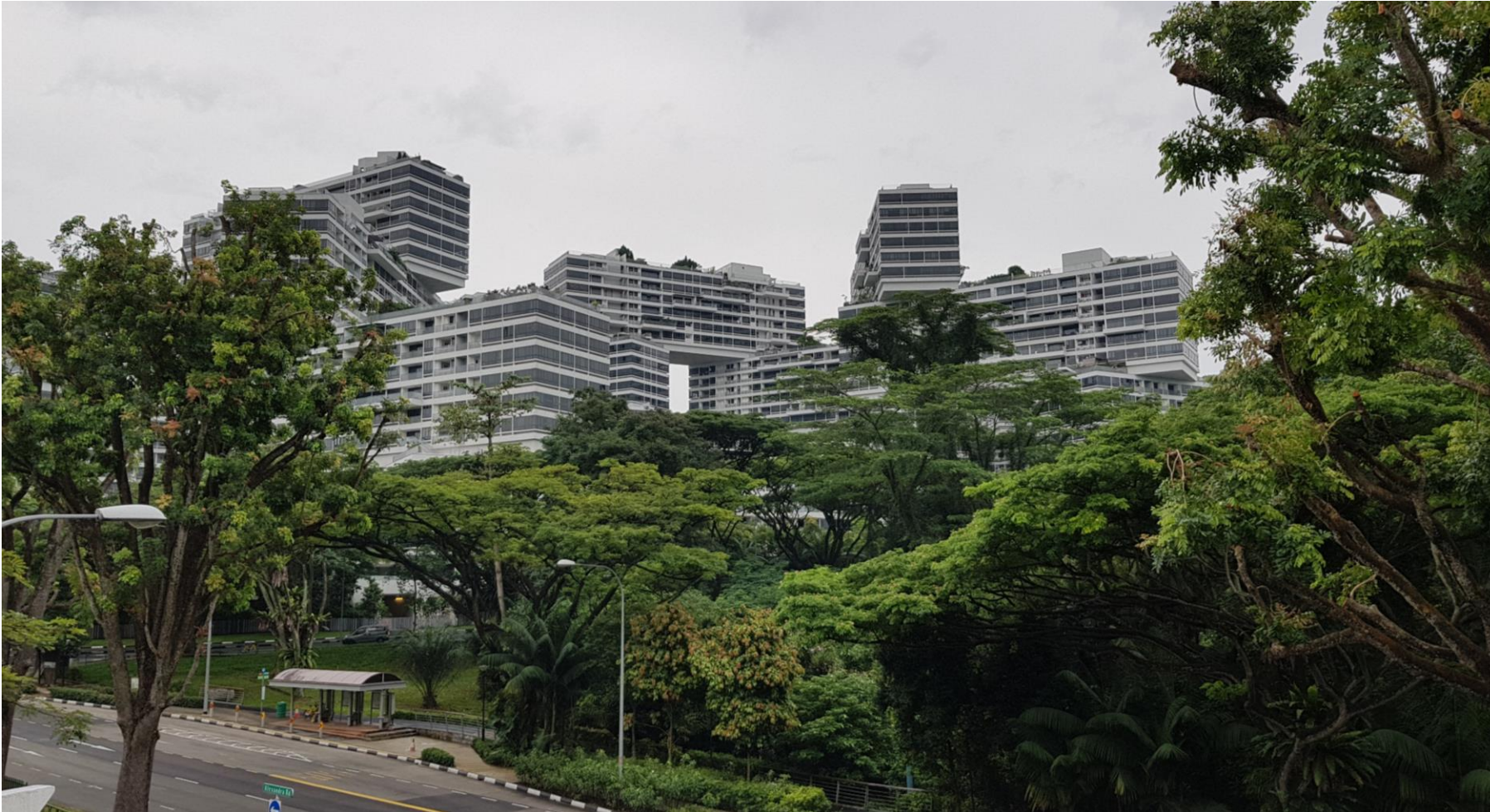
The Interlace, Singapore. An apartment complex next to the Southern Ridges Trail and features rooftop gardens, green communal areas create and garden courtyards.
