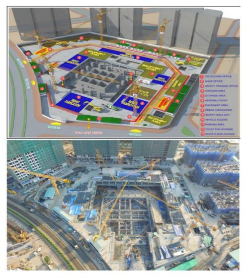
Figure 7.9 Site arrangement simulated by BIM tools (documentation shared by company C<sub>2</sub>)
