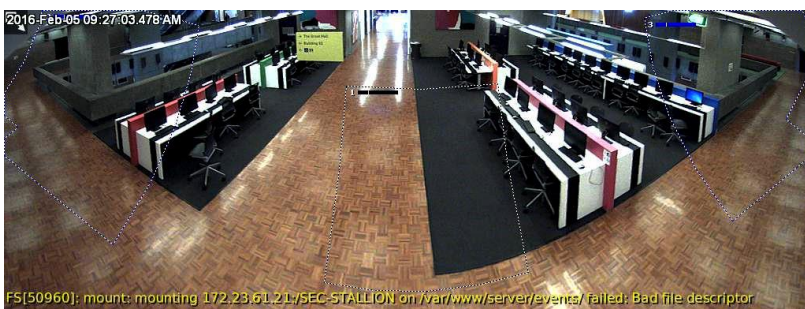
(i) CCTV Camera 9
