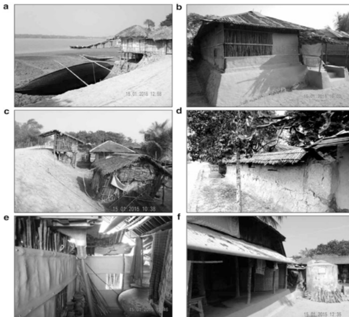
Fig. 21.3 Examples of grassroots technologies observed in Gabura. (a) Tying down boats to secure from storm surge; (b) Raised plinth height of the houses; (c) Tethering to secure house roofs; (d) Protection of mud walls from rainfall; (e) Plumbing modified to allow upstairs toilet during flooding; and, (f) Tanks for rainwater harvesting as drinking purpose
