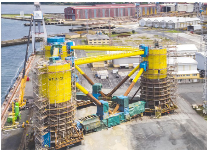
Figure 9: Semi-submersible foundation under construction at port. (Wind Europe, 2020) (Photo: Navantia)
