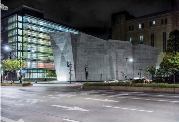
Figure 1. Spring Street Salt. Shed Photo by Ken Ohyama, CC-BY-SA
