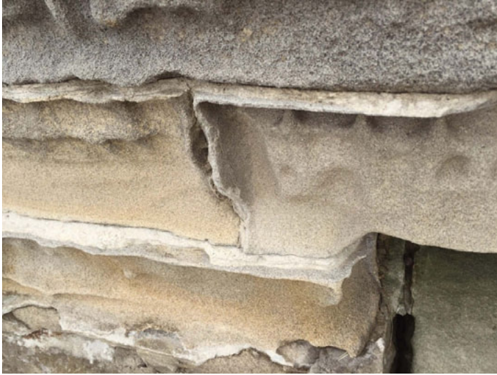
Figure 5. Sandstone blocks shown ‘withdrawing’, via erosion, from the cement mortar (Denis Byrne 2015).
