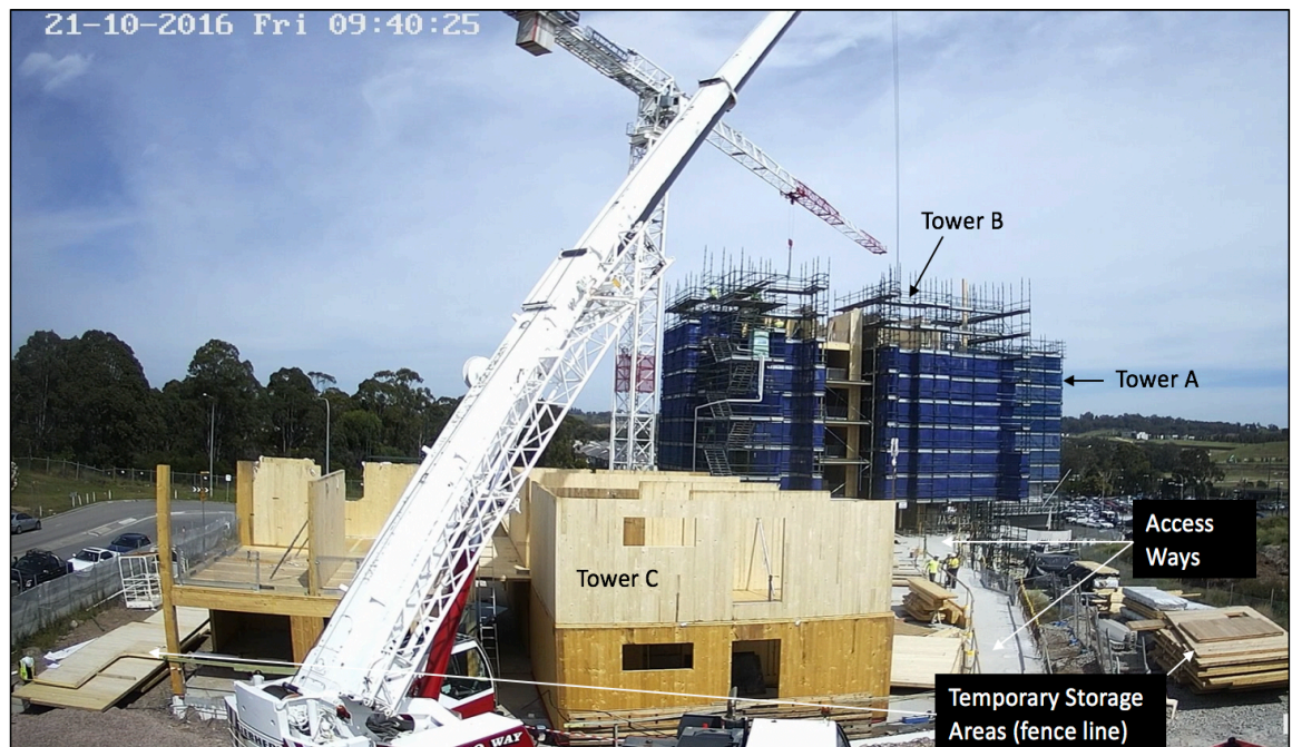
Figure 8.6 Tower C limited CLT storage area
