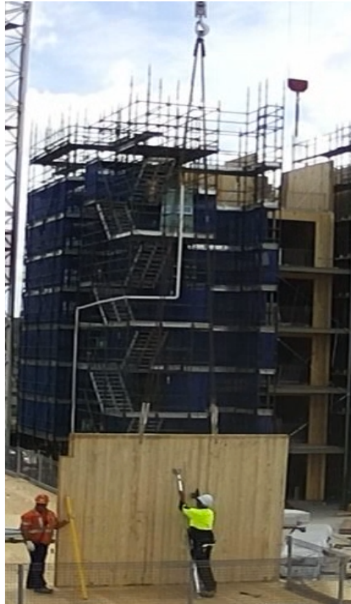
Figure 4.5 Installation of wall panel
