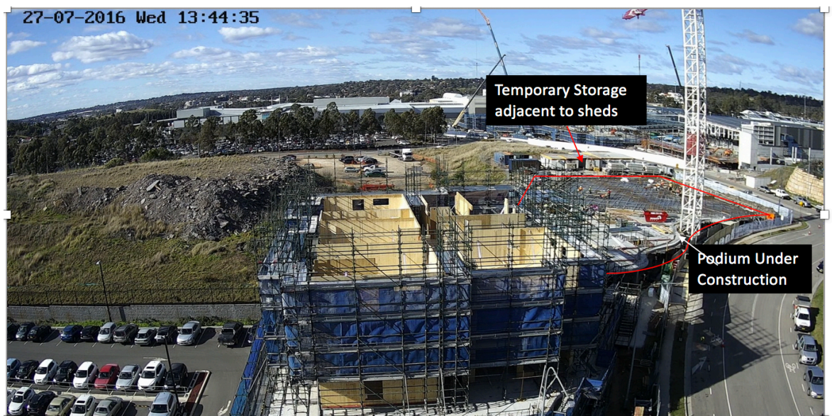
Figure 8.5 Tower A limited CLT storage area
