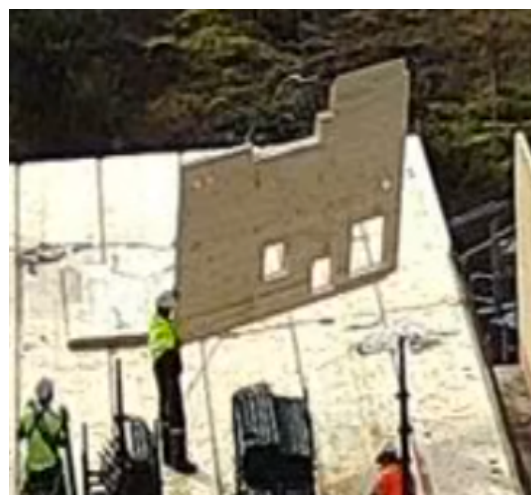
Figure 6.6 Atypical shaped (floor) panel
