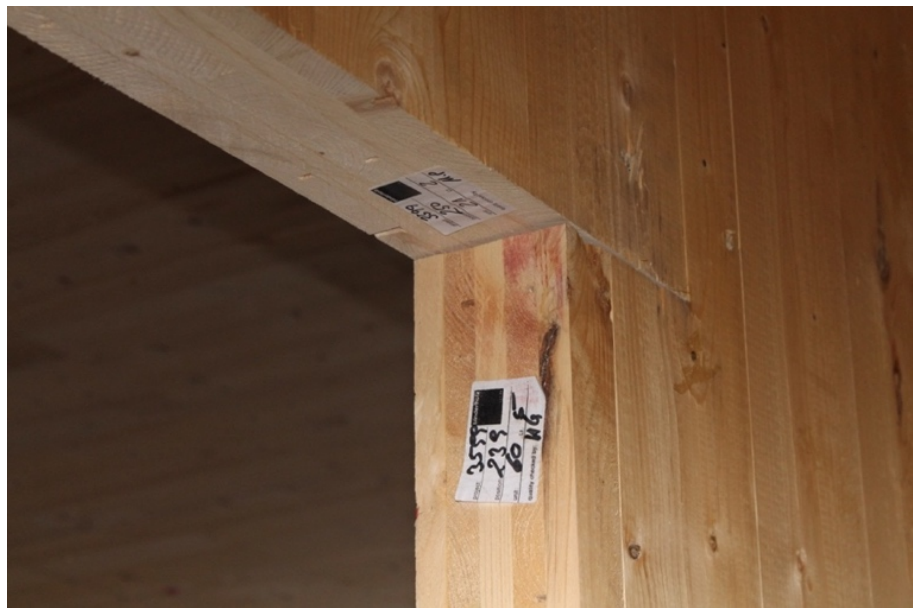
Figure 4.6 Panel ID labels attached to CLT
