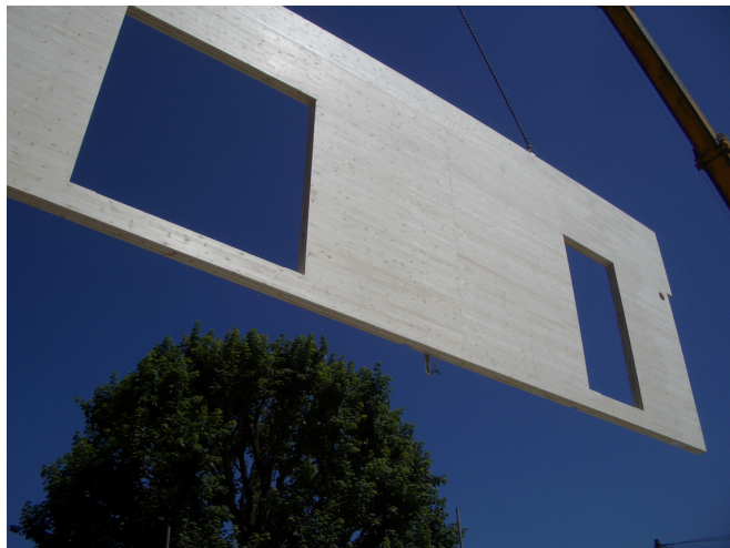
Figure 3.6 Long CLT panel with pre-cut openings craned into position
