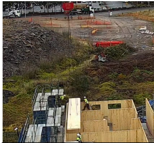
Figure 6.5 Set up point floor panel
