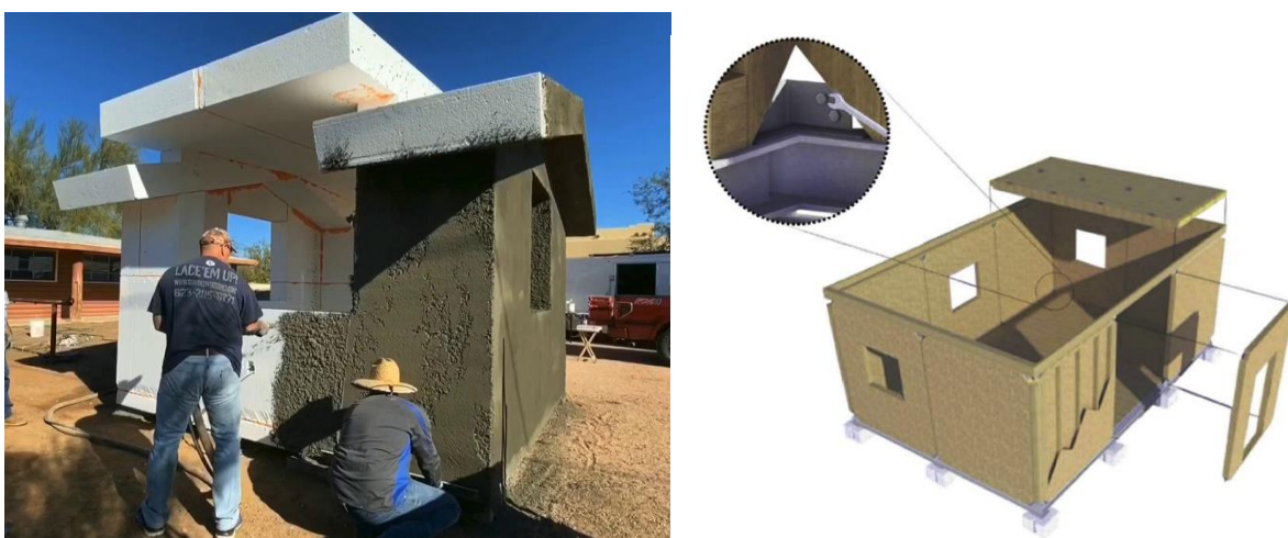
Figure 5. Left: SABS system, an innovative EPS composite structure. Right: hybrid Timber Frame (HTF) modular structure. Source: Strata International Group, Inc. (SABS 2021) and Hybrid timber wall system (Casagrande 2021)
