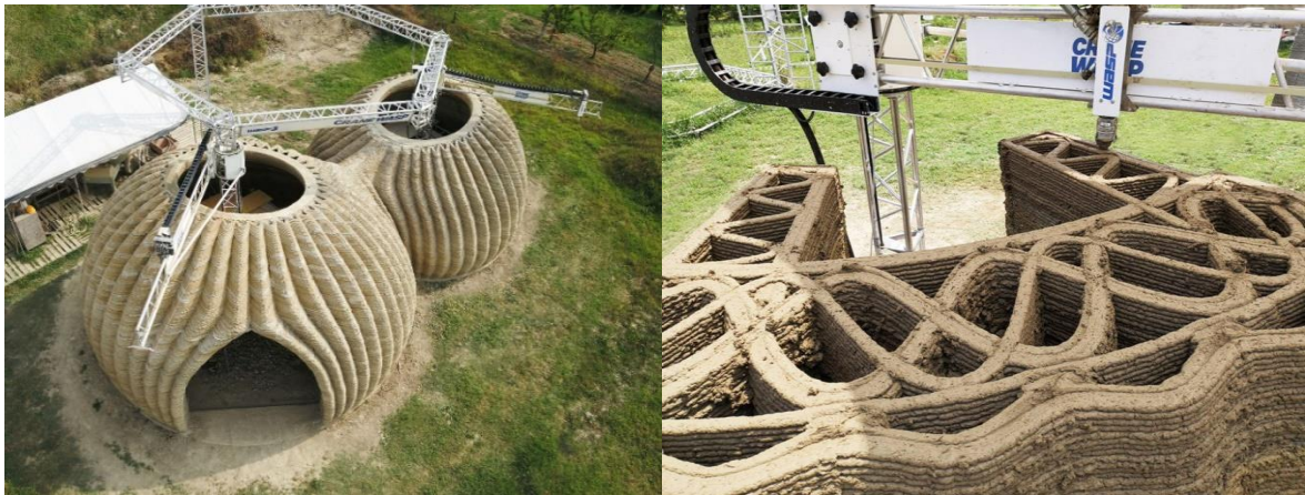
Figure 3. 3D printed structure using local resources.
