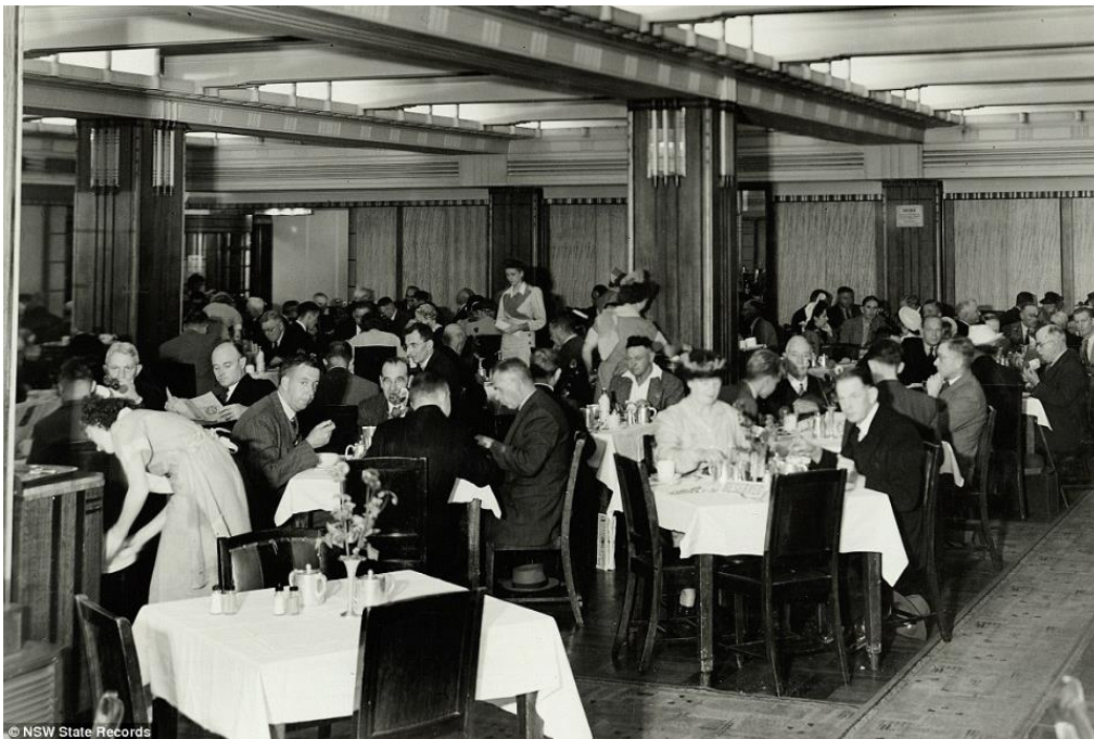
Figure 1.07 - One of the grand dining spaces constructed as part of Wynyard Station.
