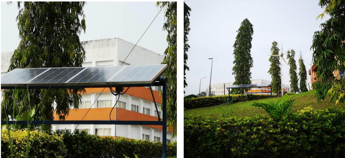
Figure 8: Photographs of the solar-assisted cooling study
