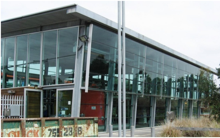
a. Water reclamation centre
