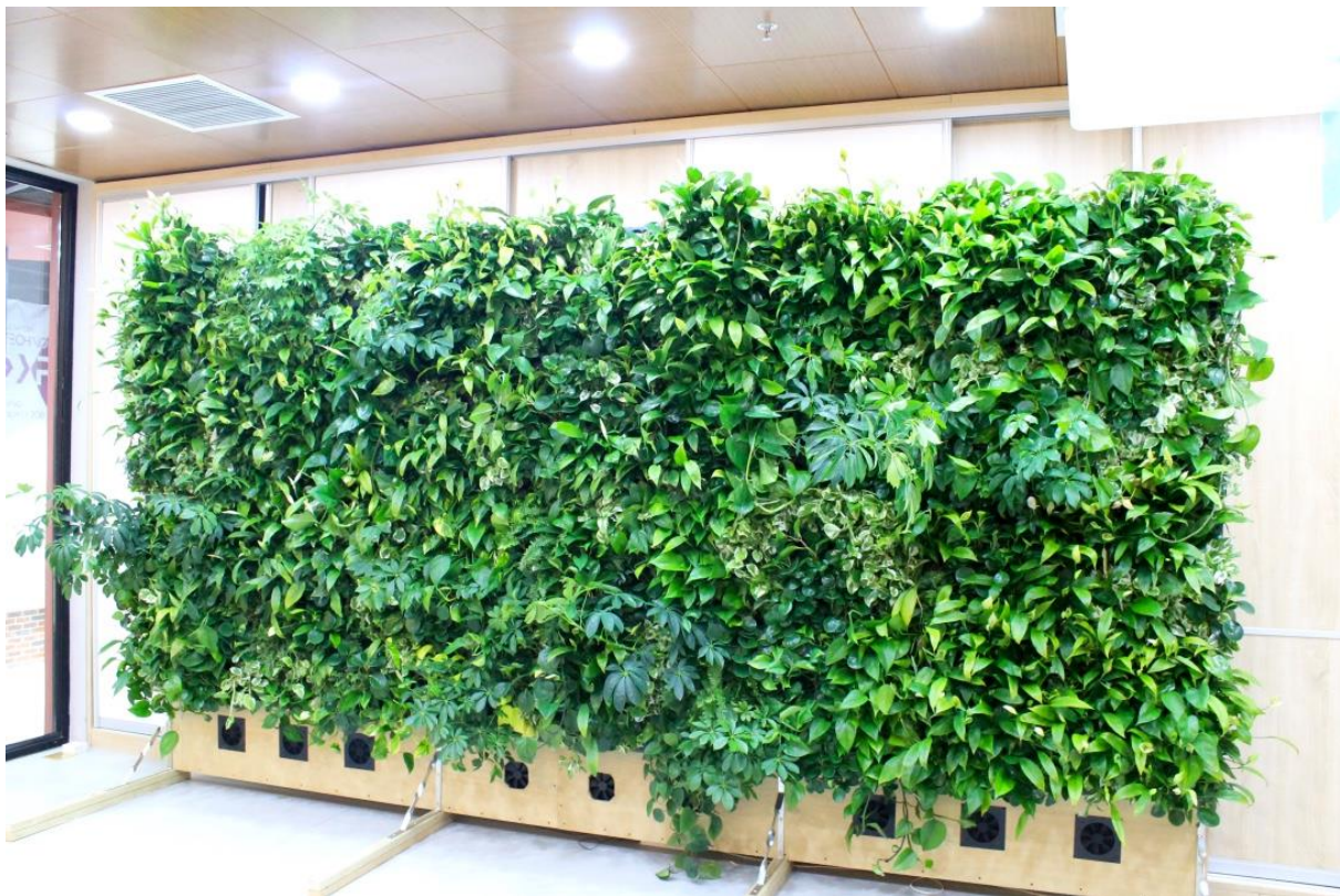
Figure 10. The active green wall used to filter ambient PM and VOCs installed in a classroom in Beijing, China.
