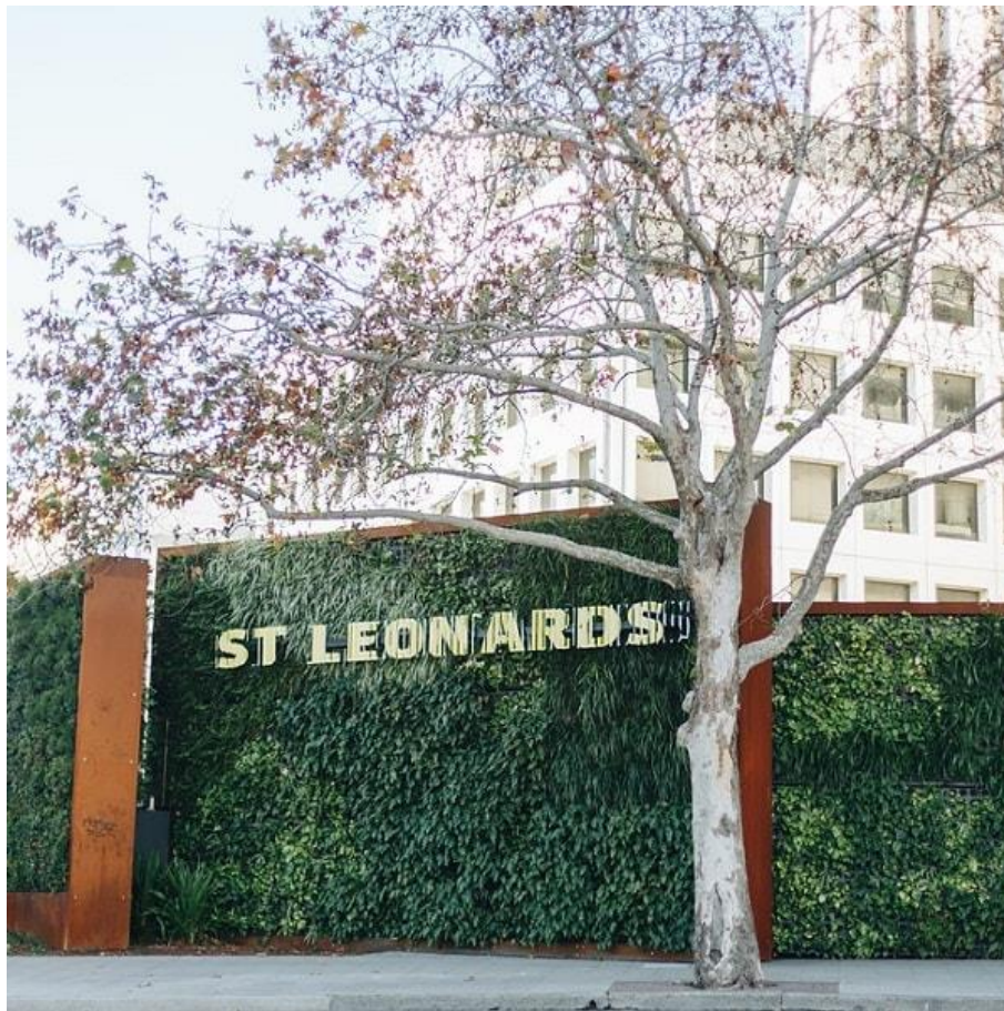
Figure 35. An outdoor active green wall (Junglefy Breathing Wall™) installed by Junglefy, in St Leonards, NSW, Australia. Figure from Junglefy (2018).
