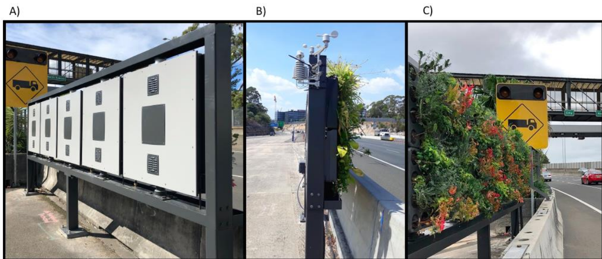
Figure 27. A botanical biofilter array. A) the rear view of a biofilter array showing five plenums arranged horizontally to form a 5 m 2 active green wall; B) a side view of the support structure with biofilter modules attached to the plenum; C) the front face of the biofilter array.
