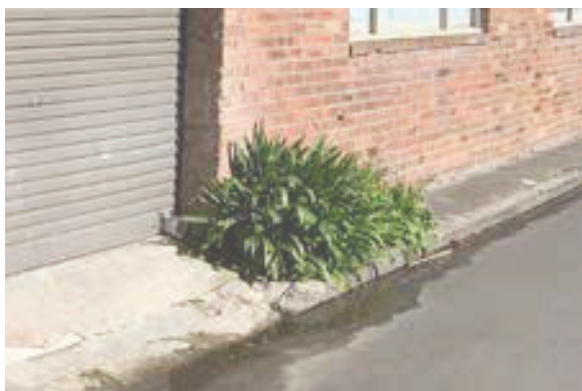
Fig. 07.05.01 Unplanned vegetation as seen down a service alleyway on-site, off of Willoughby Rd, Willoughby. Source: Author
