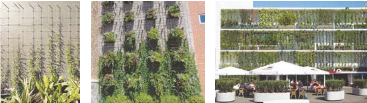
Fig. 07.05.11 Steel cable, trellis, and plant container green wall implementations. Source: [Left] Jakob Rope Systems (n/d), [Middle] Tournesol Siteworks (n/d), [Right] Jakob Rope Systems (2013).
