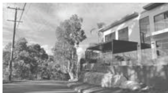
Fig. 05.01.01 A diversity of urban and suburban streetscapes and built form typologies throughout the Willoughby LGA. Chatswood CBD [Top], light industrial in East Chatswood [Middle], residential in Castlecrag [Bottom]. Source: Author.
