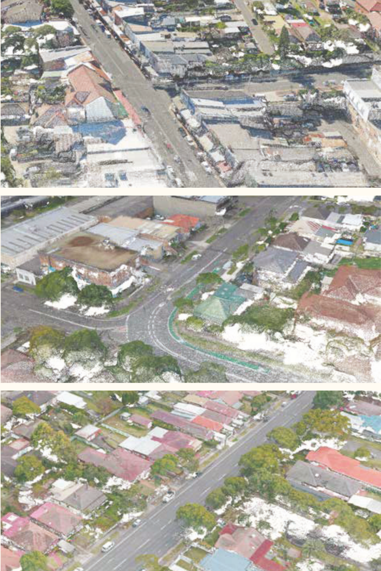
Fig. 06.03.02 Detailed views of the 3D point cloud spatial data generated from DroneDeploy, enabling numerous potentials for urban analysis, simulation, and representation. [Top] Willoughby Rd, Willoughby. [Middle] High St, East Chatswood. [Bottom] Penshurst/Royal St, Chatswood.
