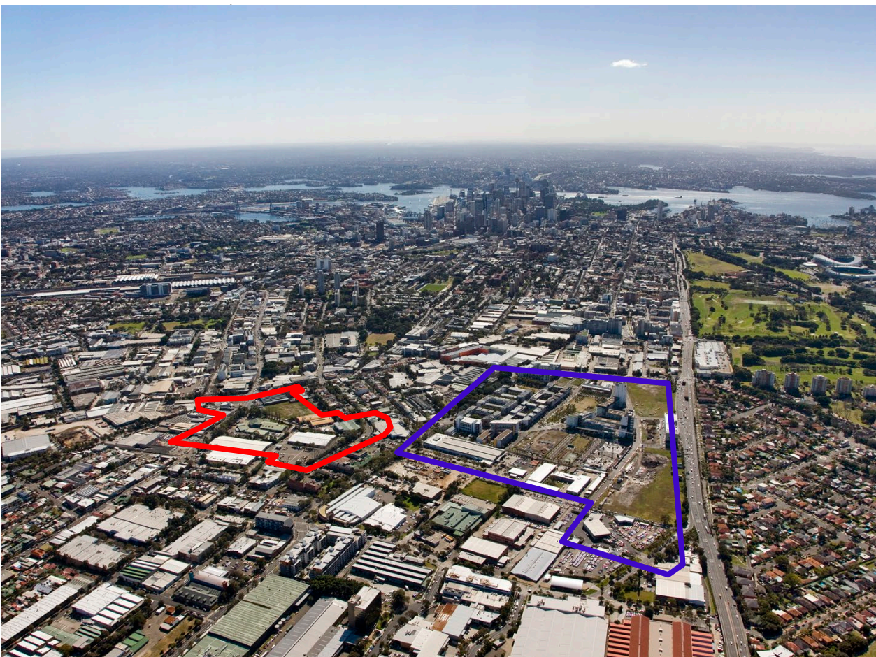
Figure 2.1: Delineation and context of Victoria Park (in blue) and the Green Square
