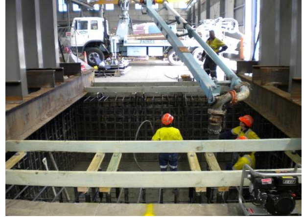
(b) Reinforced concrete of the test pit
