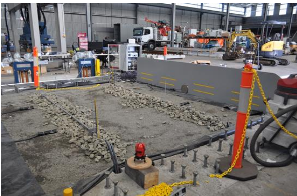
(c) Placement of ballast
