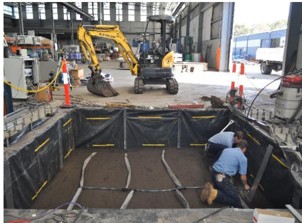
(c) Irrigation system
