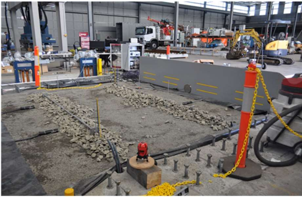
(c) Placement of ballast
