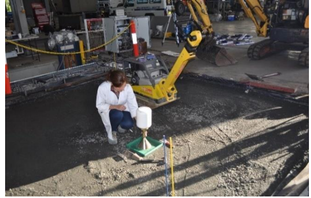
(b) Sand-cone test for compacted capping
