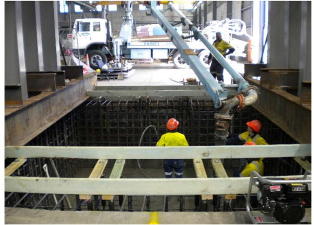
(b) Reinforced concrete of the test pit
