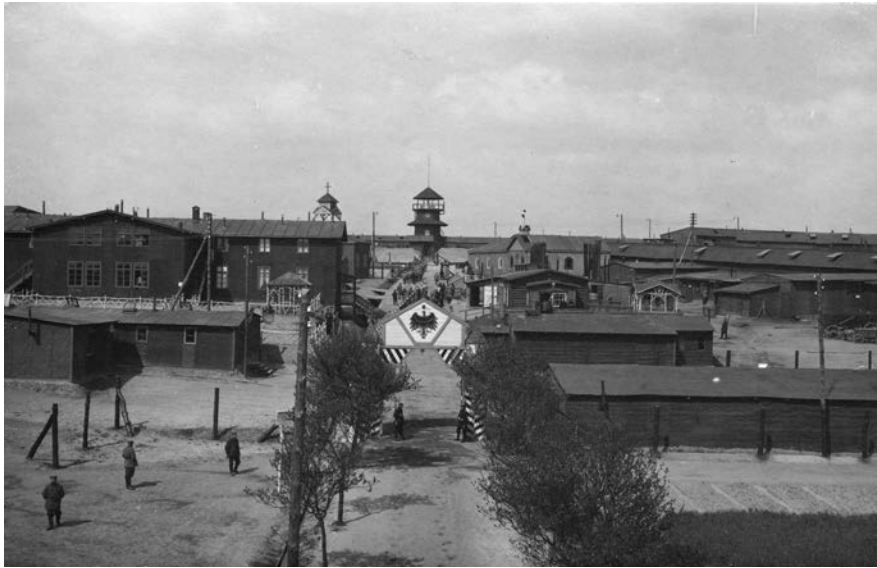
Figure 2.2: One of the prisoner-of-war camps in Crossen constructed using the Kruchen System. © Bundesarchiv R 67 Bild-02-002.
