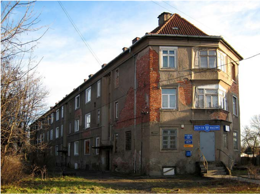
Figure 2.5: The end of the bar building, Siedlung Bunte Reihe. The angling of the facade to animate the building end and the brick construction are both apparent here. © Creative Commons.
