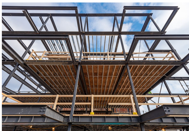
Fig. 1: Typical cold-formed steel and timber composite floor under construction.
