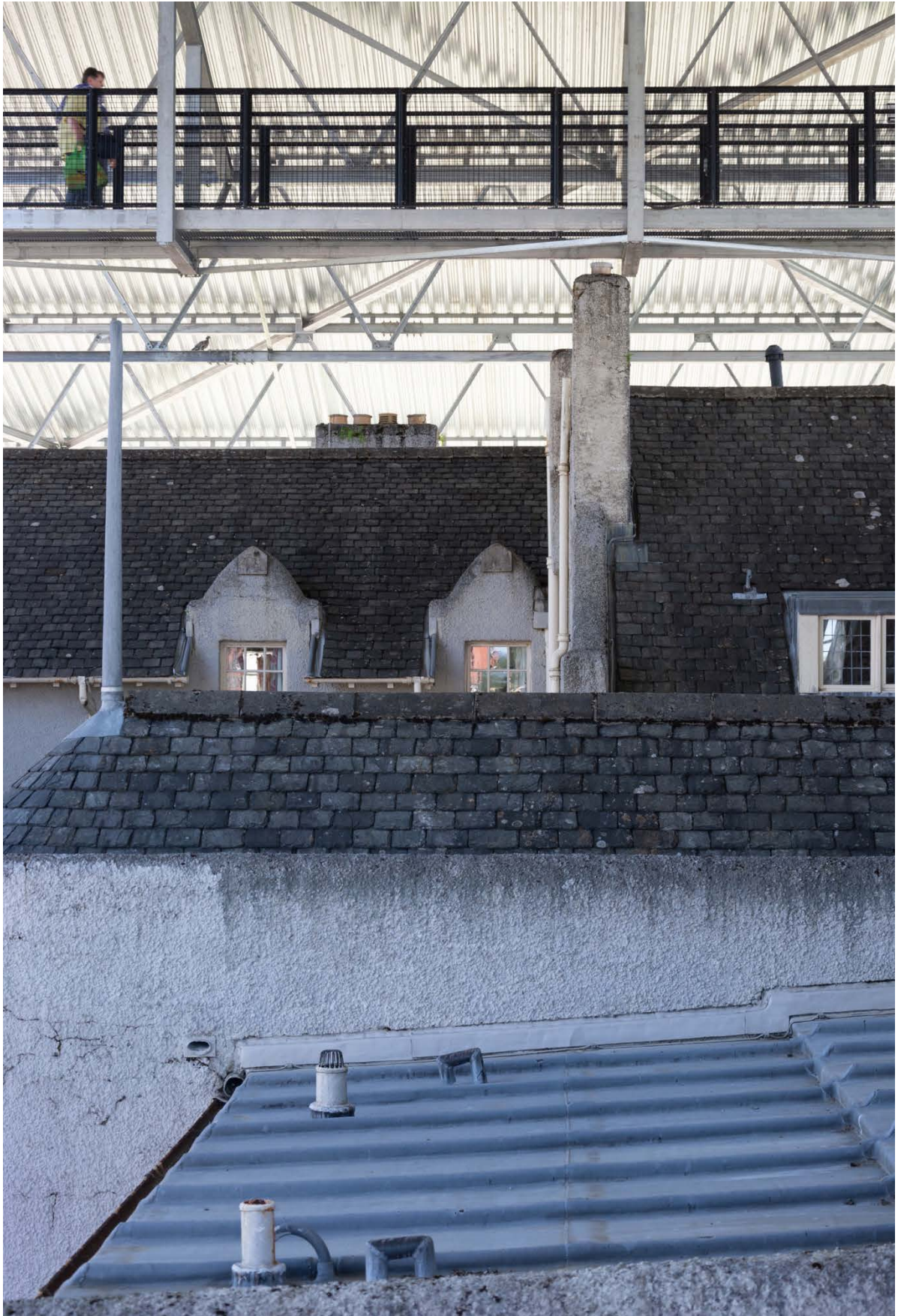
Figure 18. One of the walkways crosses over above the roof of the house, 2019
