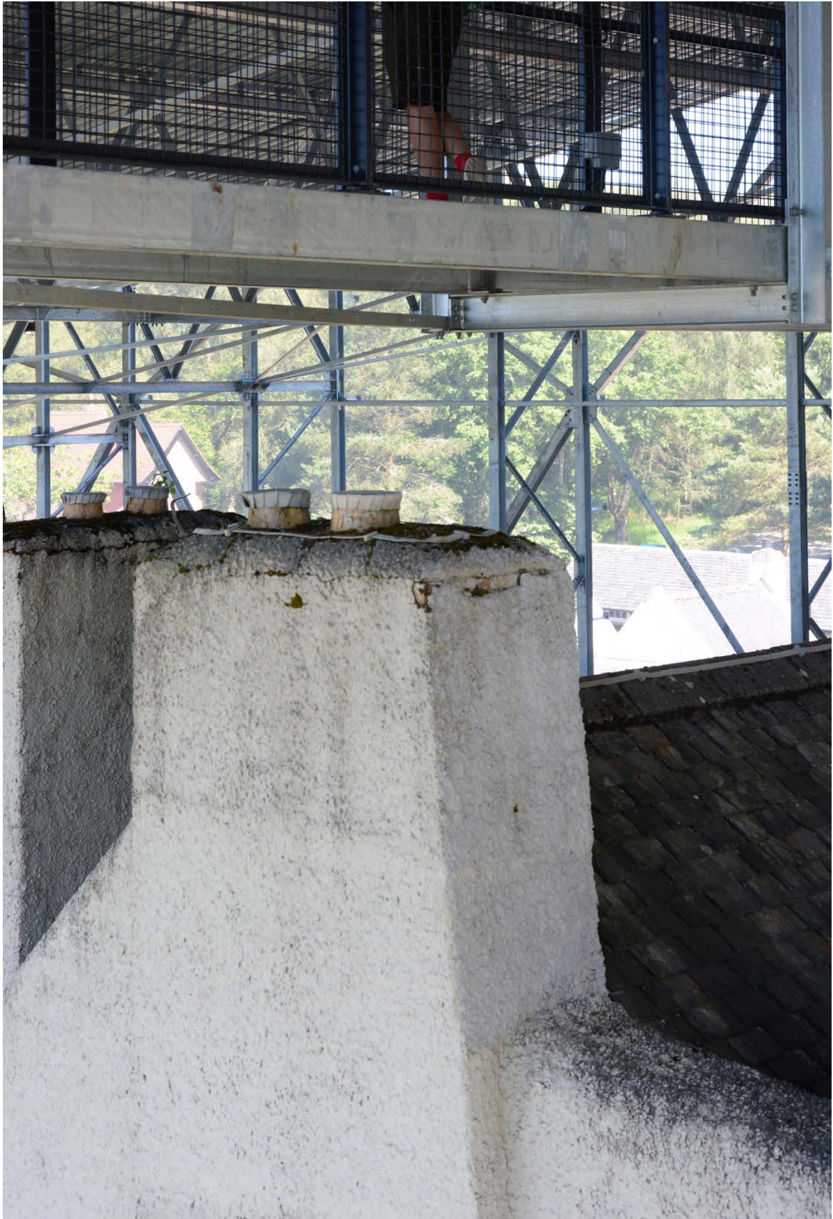
Figure 19. The walkway above the chimneys, 2019
