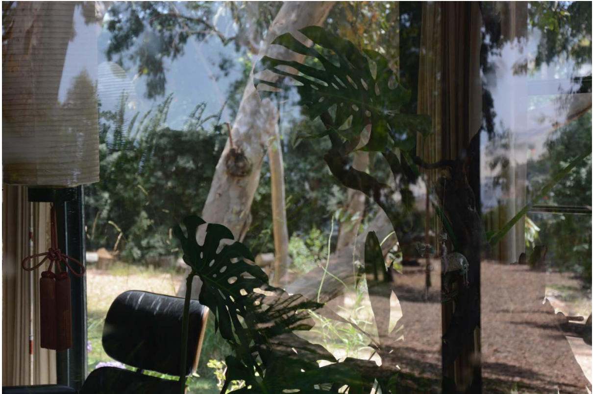
Figure 23. The reflection on the glass walls obscures the interior view, 2019
