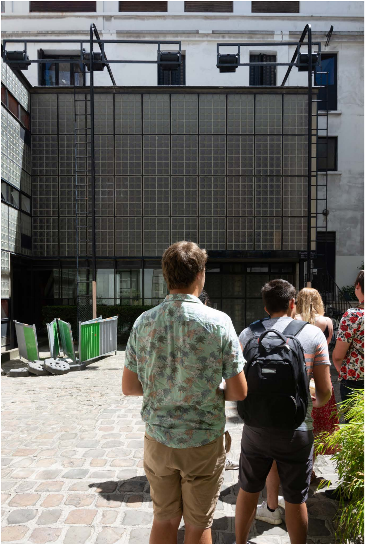
Figure 30. The facade from the courtyard, 2019
