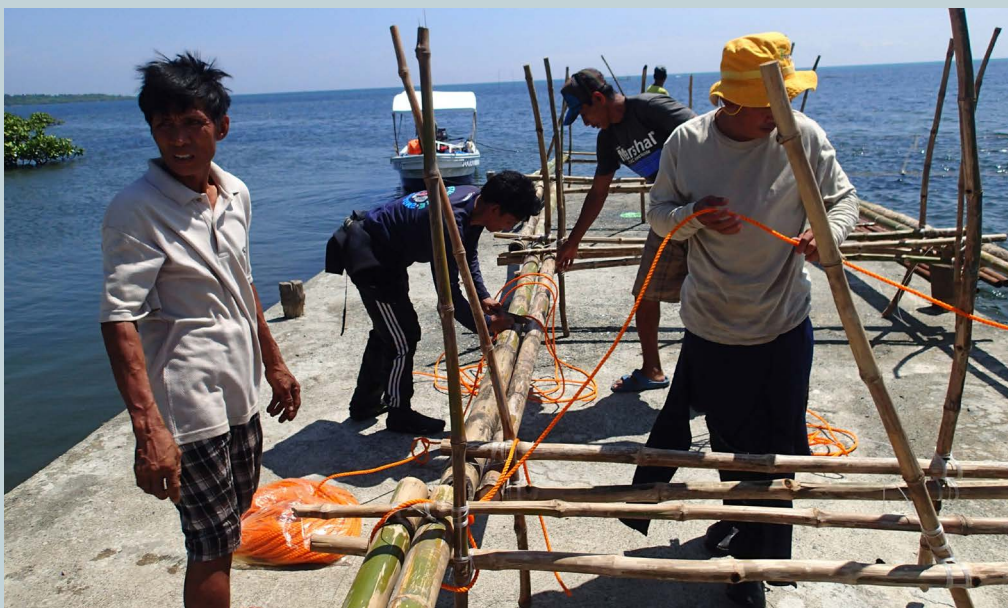
Figure 23 Construction of floating hapa bamboo frames at Imbo
