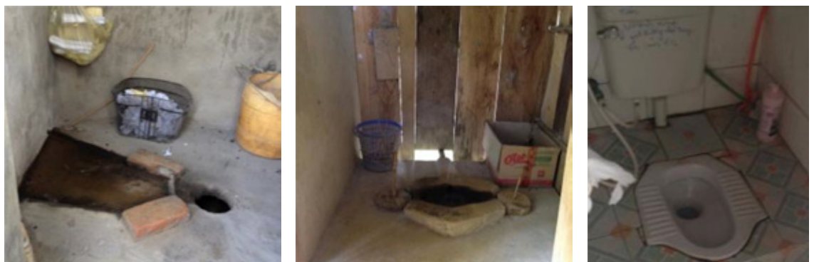
FIGURE 4 VARIATIONS IN TOILET MODELS – FROM LEFT TO RIGHT: PIT LATRINE, DOUBLE VAULT LATRINE AND SEPTIC TANK LATRINE
