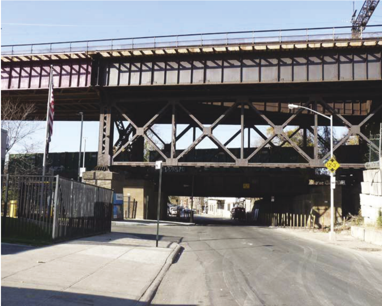
Figure 10 The South Bronx access point to the Randalls Island Connector as yet has no obvious signage to direct pedestrians or bicyclists (Walsh 2016)
