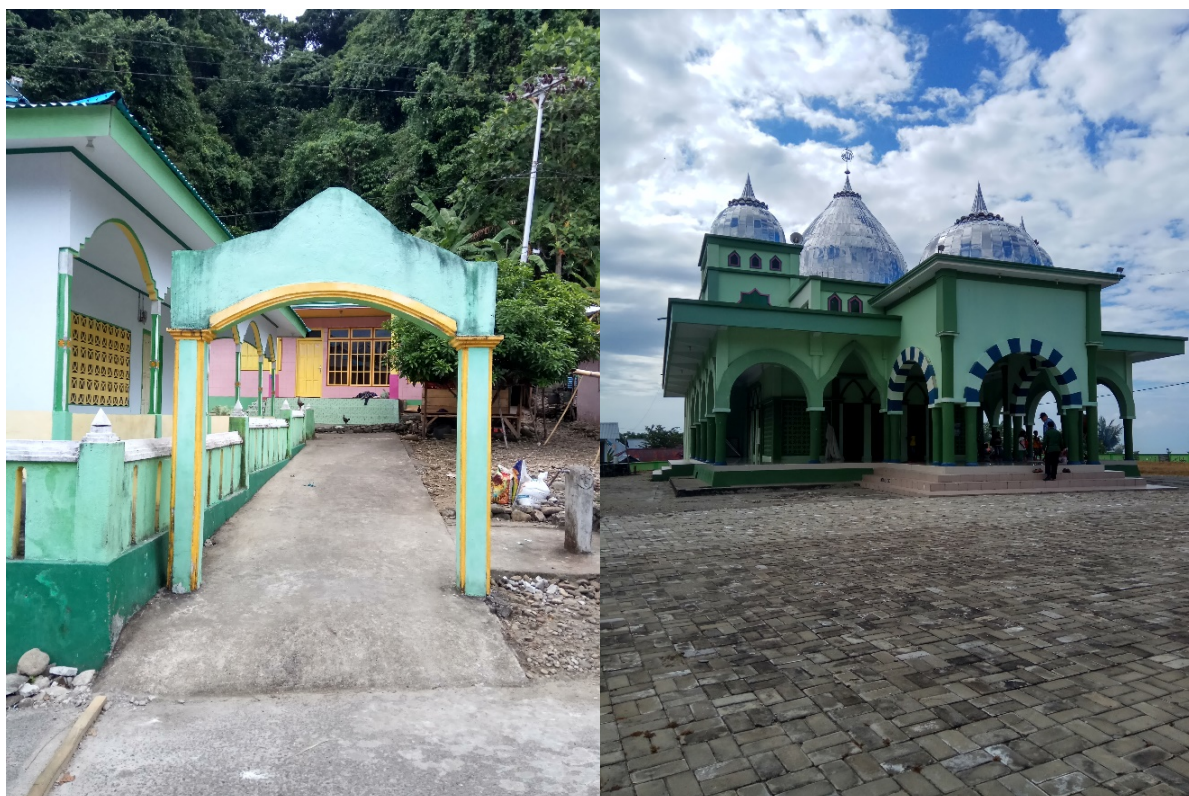
Figure 15. (L) A mosque entrance on Ambon Island repaired and concreted using Premium Fund finances. (R) A mosque on Buru Island which had flood damage of a retaining wall repaired using Premium Fund finances (Photos: Dedi S. Adhuri).
