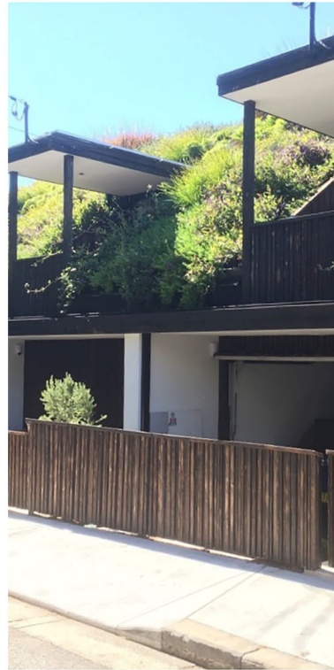
Green roof on sloping roof in Sydney, Australia (Photo by: Author)
