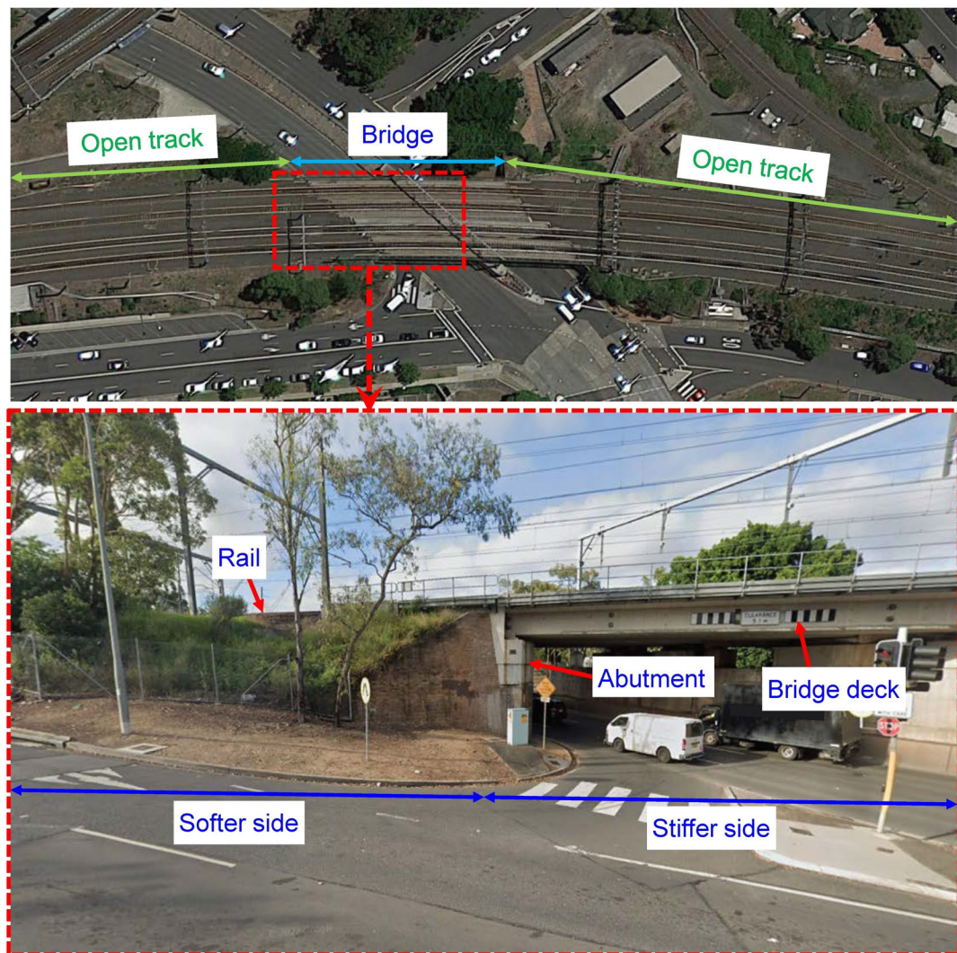
Figure 1.2 Open track-bridge transition [Imagery © 2022 Google, Imagery © 2022 CNES / Airbus, Maxar Technologies, Map data © 2022; Image: © 2022 Google]
