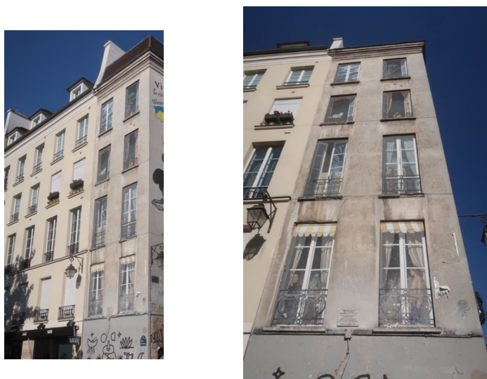
Figure 2. An example of a trompe-l'œil painting emulating a façade with windows (the two rows of windows on the right are not real, as can be seen in the close-up in the right image). This is on a building near the Centre Pompidou in Paris.
