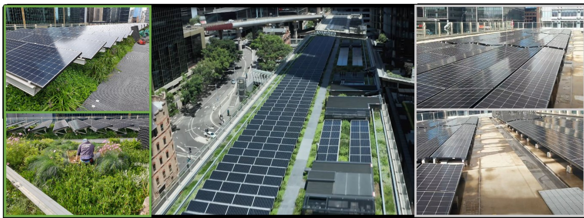
Figure 1. Aerial image of the study site (centre image). Daramu House (bio-solar; left two panels) and International House (conventional solar; right two panels). Sister buildings were near-identical with the exception of roof surface cover (plant material vs concrete). Plant material covers all regions of below panel areas on the bio-solar roof.
