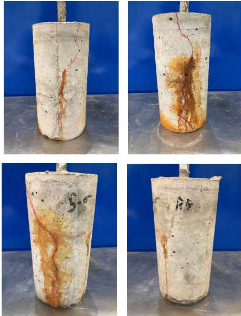
Figure 4-20 Cover cracking of cylindrical specimens embedded with N12 rebar outlined with red colour
