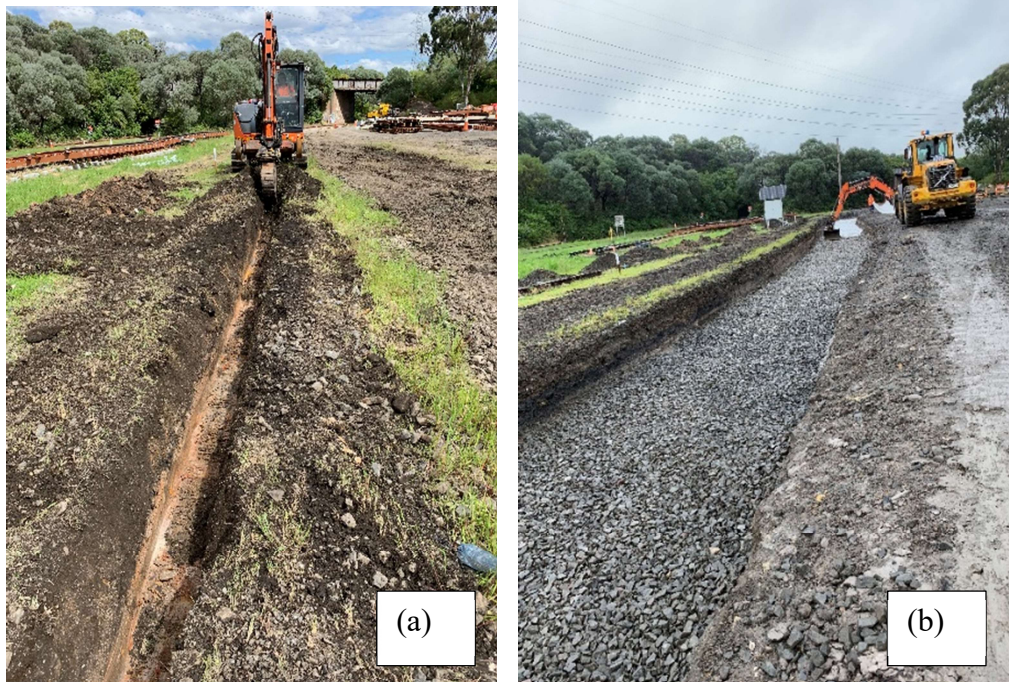
Figure 8.4 Ground preparation (a) excavation starts from the centreline of the track, and (b) the drainage layer on top of the subgrade is separated by a non-woven geotextile
