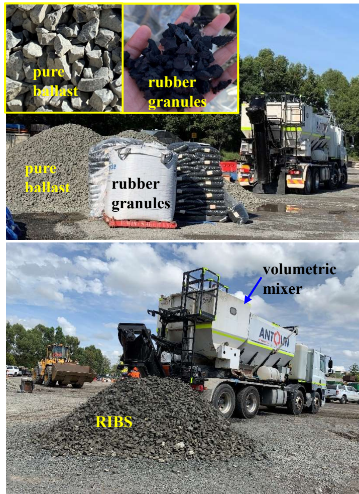
Figure 8.3 Mixing the ballast and rubber granules at the site (a) the materials before mixing, and (b) volumetric mixer while producing RIBS
