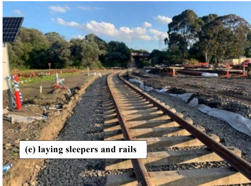
Figure 8.8 Stages of RIBS track construction
