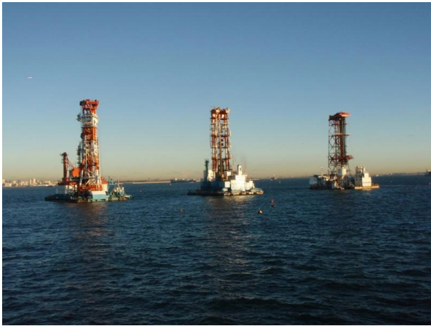
Figure 14: DMM vessels in operation (Courtesy of the Tokyo/Haneda International Airport Construction Office).
