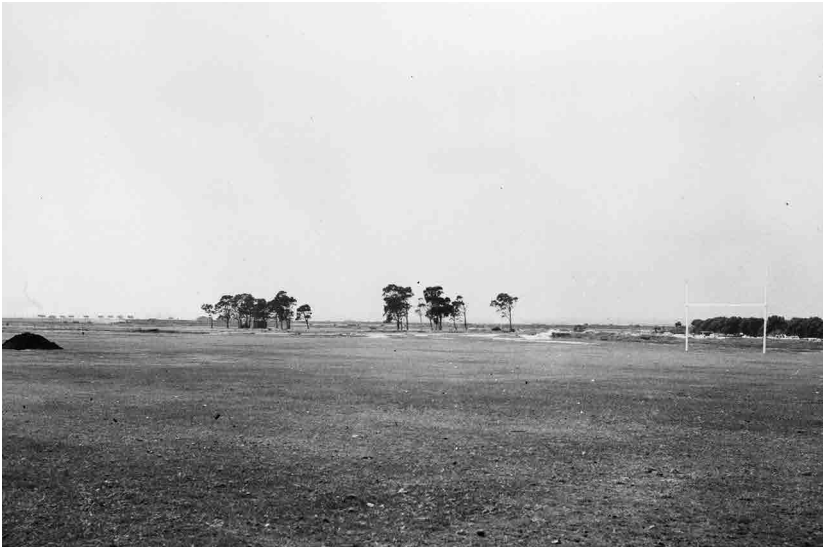
Figure 7.4: Goal posts erected after swamp ‘clearance’.
