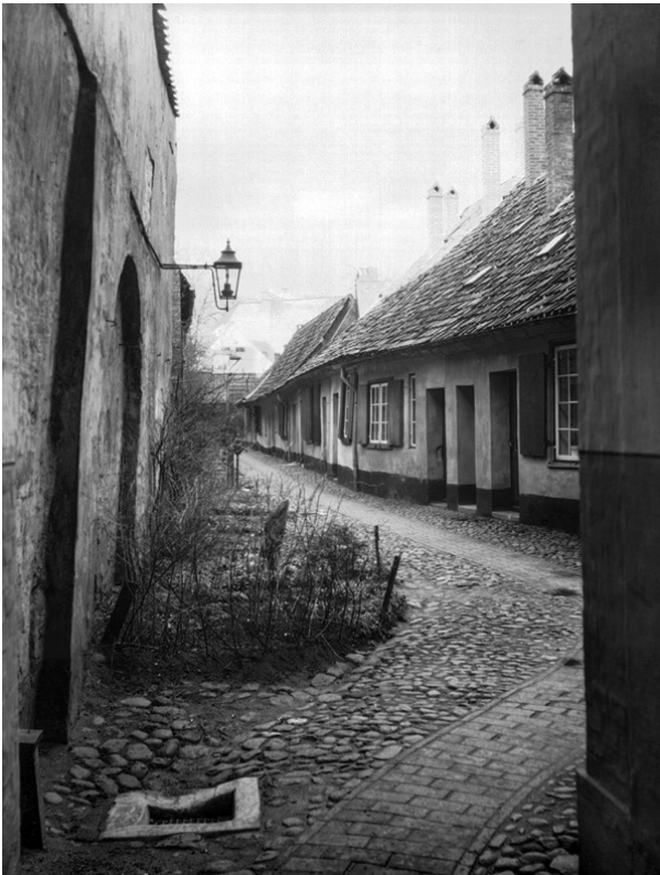
Figure 1. Residential lane off Glockengießerstraße 41–3, Lübeck, constructed in 1612. Source: “Gandorps Gang – Hof” [Gandorps Gang – Courtyard] (1925), © Bildarchiv Foto Marburg.
