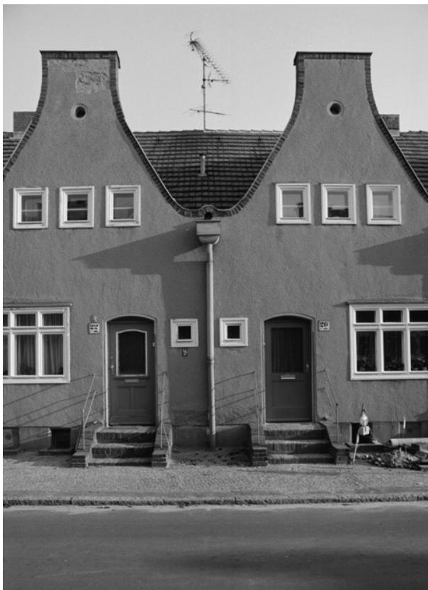
Figure 9. Schmitthenner's housing on the street "Zwischen den Giebeln" in the Staaken garden city, Spandau, Berlin. Source: Vorsteher (1978), © Bildarchiv Foto Marburg/Dieter Vorsteher.
