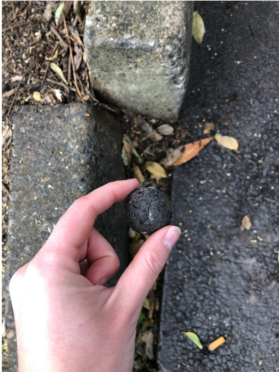
Figure 15: Working with cracks, 2019. Digital photograph, © Mapping Edges.
