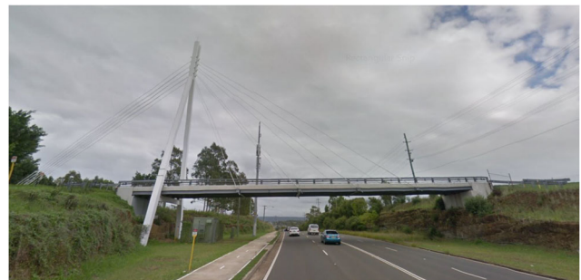
Fig. 4 The cable-stayed bridge from our first case study, Western Sydney, Australia (source: Google Earth)
