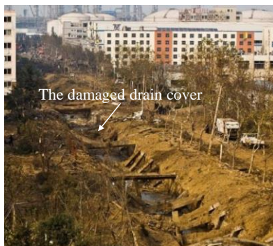
Fig. 1 The explosion site in Qingdao (Hou et al., 2021)
